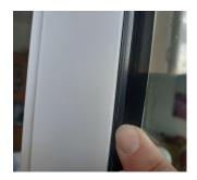
Start at the edge of the window. Remove the liner with one hand and attach the edge sealing tape with the other hand partly onto the window film and partly onto the glass pane for a good sealing result.
