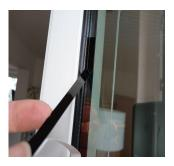
If you need to adjust the edge sealing you can lift Apply the Avery Dennison<sup>®</sup> Edge Sealing Tape the tape up and readjust it.
